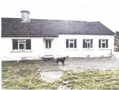
Chimney Front View
