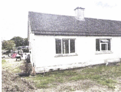
Chimney Front - side view
