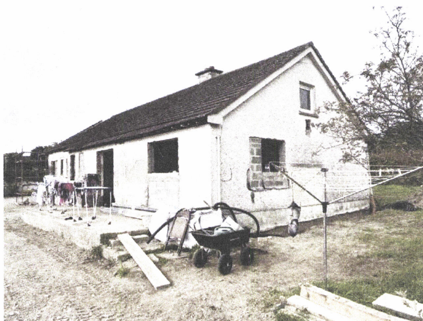
North East view – Utility will sit where the large gravel bags are
