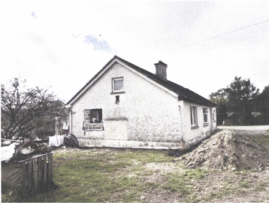
Bifold door wall view, side profile of Chimney
