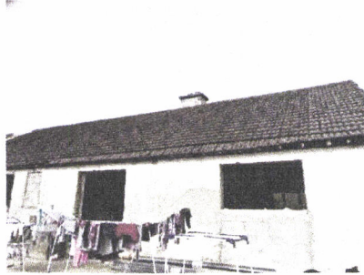
Chimney rear view
